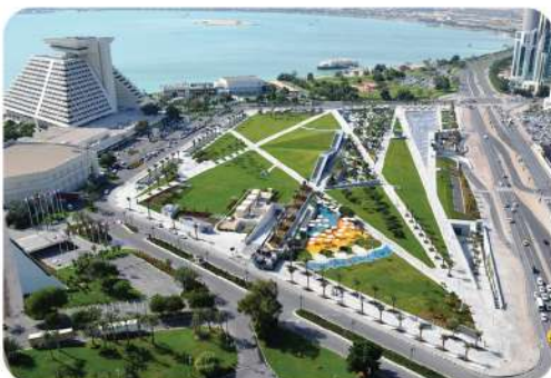
Sheraton Park Project Qatar
